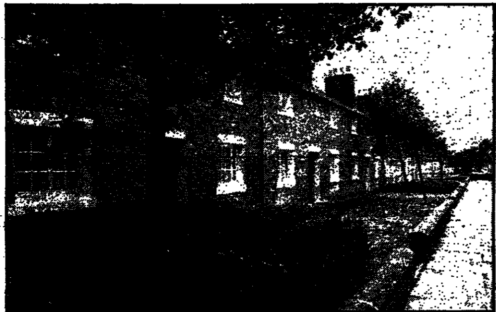
The renovated Railway Village housing is a Swindon landmark
